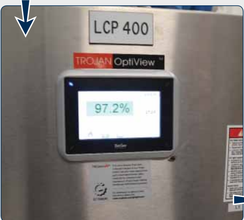
Water is then treated with ultraviolet light to deactivate any remaining organisms. The UV light transmission display provides an accurate assessment of how pure the water is.
