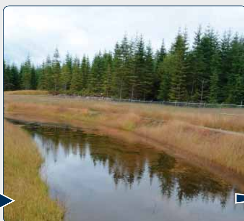
Waste water is pumped to one of two settling ponds onsite. Though slightly sandy in texture, when the waste material is dried it can be mixed with topsoil and reused for gardening.
