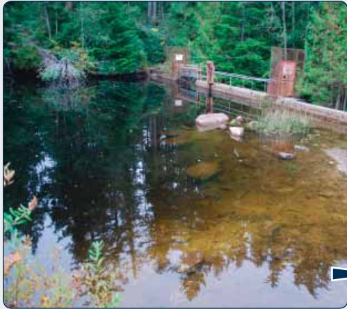
Water for the McNeill Lake treatment plant is pumped directly from the often murky lake.
