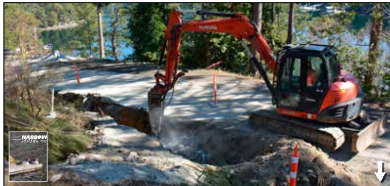
APRIL: Water system upgrades on Francis Peninsula were pushed over-budget due to unexpected amounts of bedrock.
