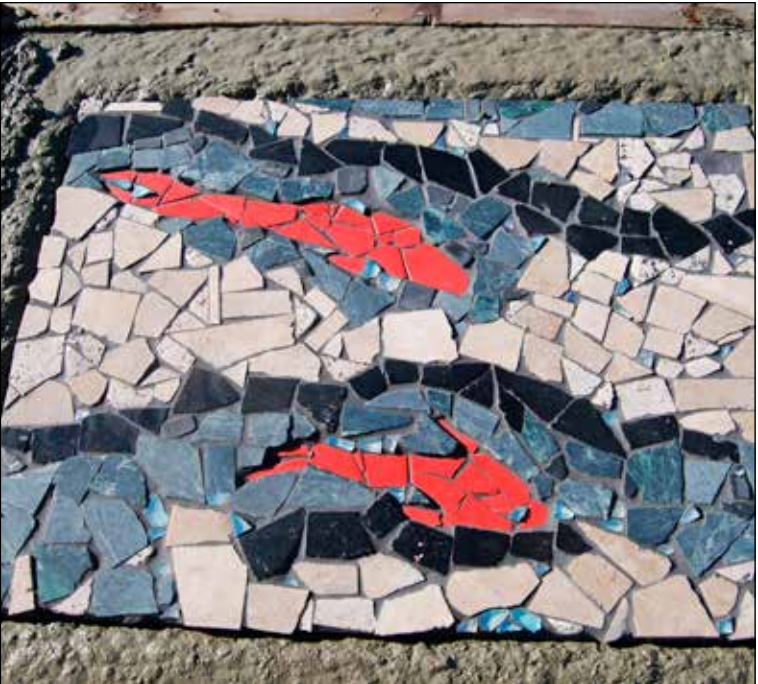
Brian Lee This mosaic has just been set into the concrete awaiting finishing. March 2021
