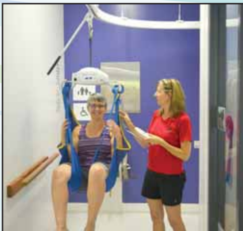
New accessibility equipment was installed at the facility June 2016.
