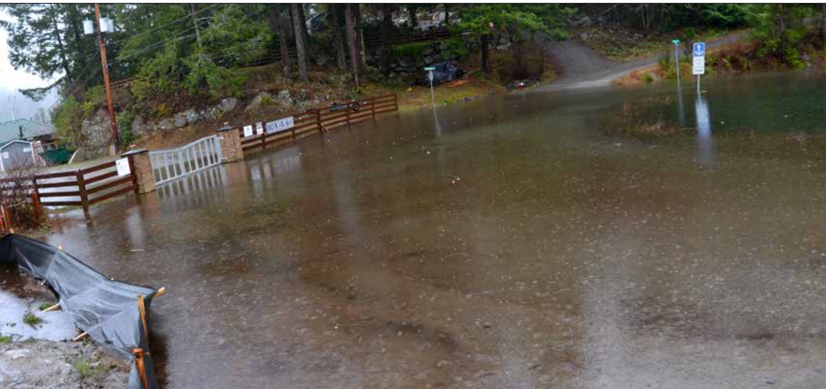
Seasonal high tides on Dec. 27 coincided with heavy rains that swelled Pender Harbour's banks in many places. The annual saltwater seen above. These photos were taken in the morning of Dec. 27, just after the peak of the 17.1-foot (5.2 m.) tide.
