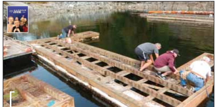
MAY: P. H. Rotary Club members volunteered their time to repair the Garden Bay Marine Park's dinghy dock last April.
