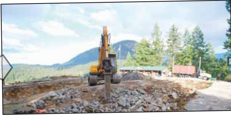
MARCH: Last remnants of the P. H. Hotel were trucked away while the site was prepared for construction of a new building.
