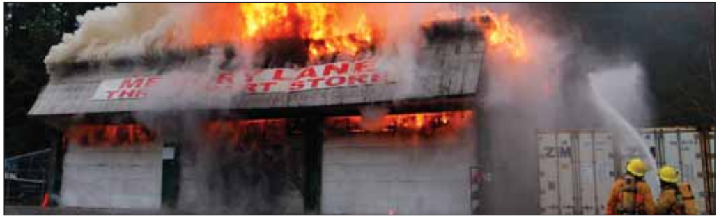
1:09 p.m. Fire breaks through the roof.
