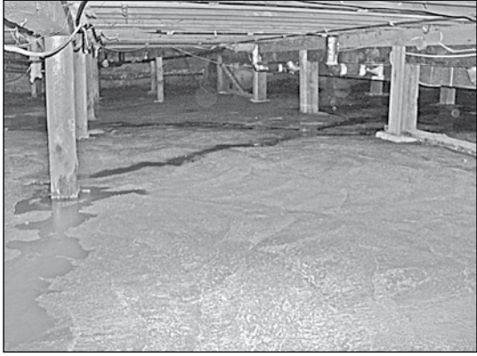
After draining the "rat poo soup", the basement of the hall now has a fresh floor of dry concrete for extra storage.
