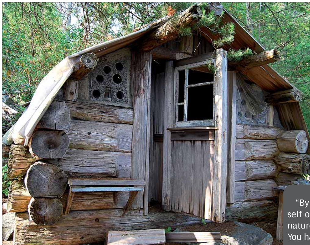
The guest cabin is slowly deteriorating from neglect but is still a fascinating piece of hand built architecture.
