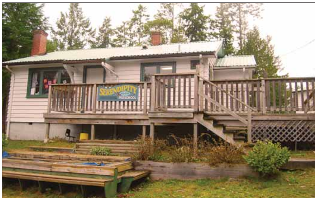
The Serendipity Child Development Society moved the preschool to this former forestry building in 1987.
