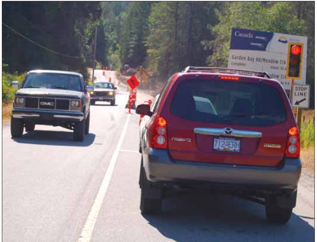
Pender Harbour's first traffic light is only temporary as crews work to replacing aging culverts with a bridge over Meadow Creek on Garden Bay Road. The project will cost just over $1 million and will be paid for by federal infrastructure stimulus funding .
