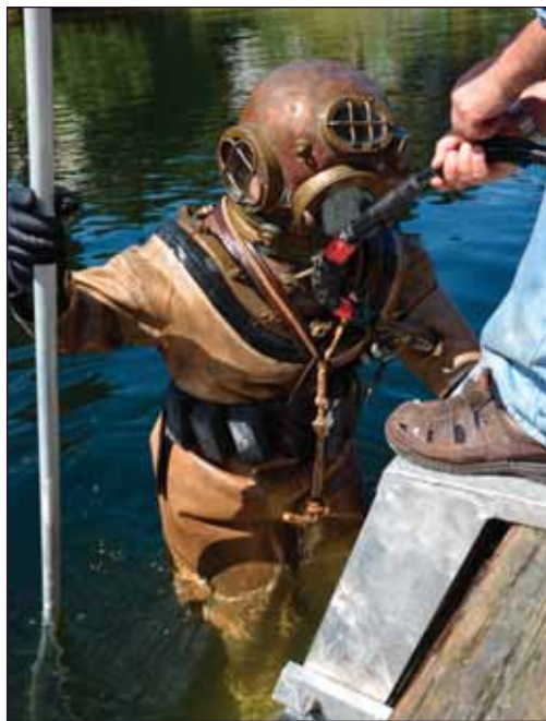
A hard hat diving demonstration on Saturday provided a live feed of the ocean floor beneath the Madeira Park government wharf docks.
