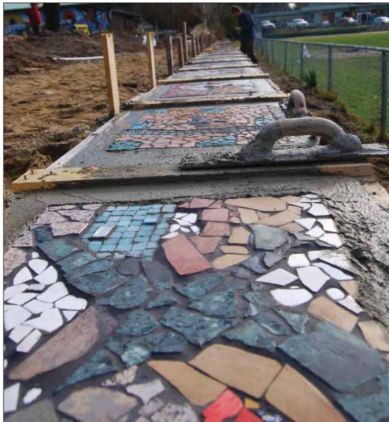
Rob Saunders adds the finishing touches to the concrete borders
