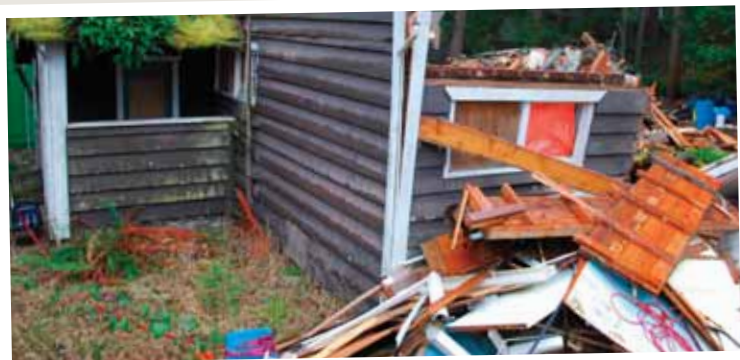
The historic 'Teachorage' building in Madeira Park was demolished on March 21.
