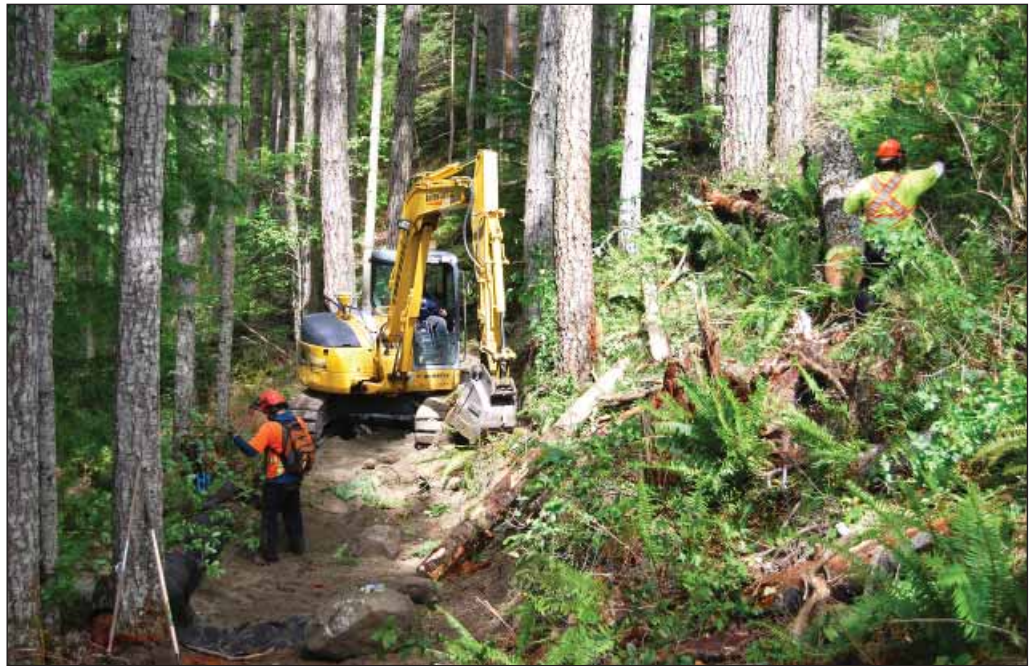
About 10 trailbuilders are working full-time to complete the Suncoaster trail by July 30. Crews break up to work in various sections simultaneously. Seen here is Andrew Curtiss blazing trail in the excavator while John Sterle and Clifford Silvey follow behind.
